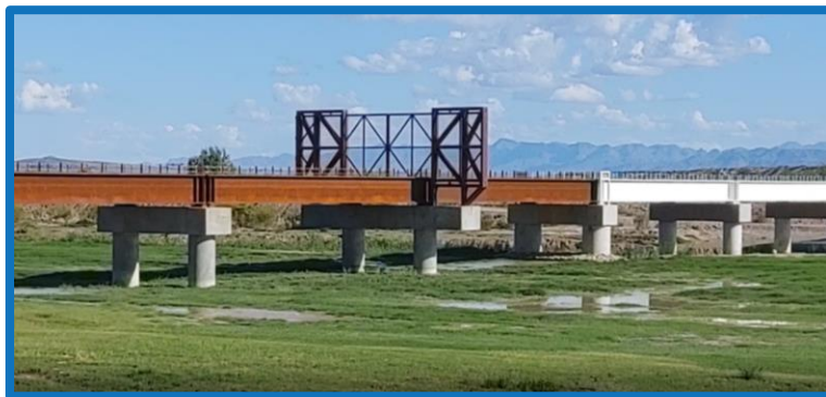
Presidio-Ojinaga International Rail Bridge in October 2019 – Scheduled for freight operation in April 2021 Credit: Brad Newton, Presidio Municipal Development District (PMDD)
