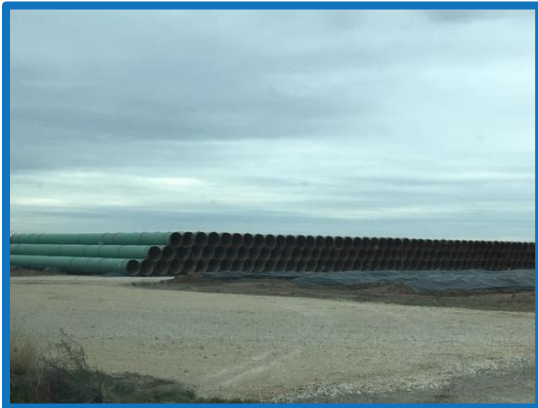
Interregional pipeline components in San Angelo
